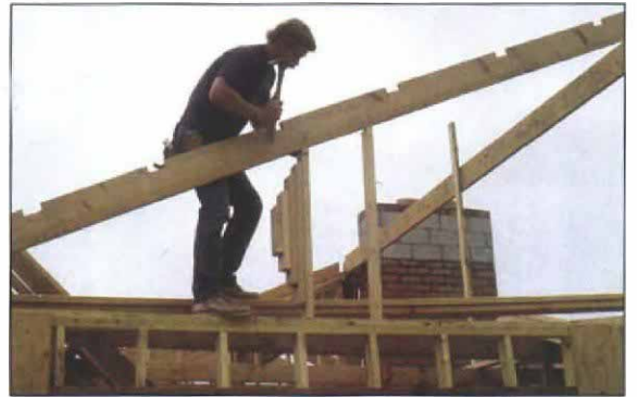
Installing the studs. Nail through the rafter into the studs to keep from putting a hump in the rafter.
